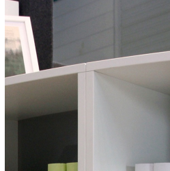
Carcass mitered tightly glued
